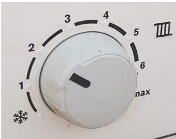
Your combi boiler will usually have one or two temperature dials on it. One will have an icon that looks like a radiator next to it — this is the dial for the "flow" temperature, which determines your radiator temperature. The other dial (if you have one) will probably have an icon of a tap next to it, and controls the temperature of your hot water (i.e. that comes out of your taps and shower). Here, you will be adjusting the flow temperature control.
